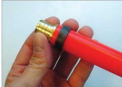
2. Slide crimp ring over end of tubing. Insert fitting into end of tubing until it stops. Position the crimp ring 1/8" to 1/4" from the end of the tubing and over the ribs of the fitting.
